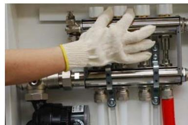
9. Filling the system: open the first lockshield by turning the Allen wrench anticlockwise.
