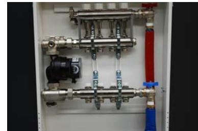
5. Connection and tightening of entry/return flow secondary circuit from high temperature and low temperature system.
