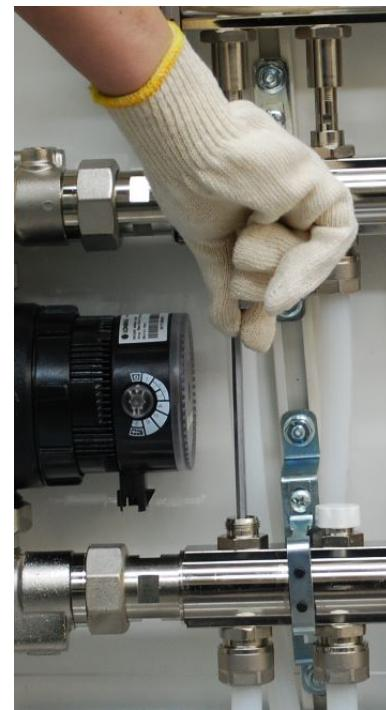
10. Filling the system: close the following lockshields by turning the Allen wrench clockwise.
