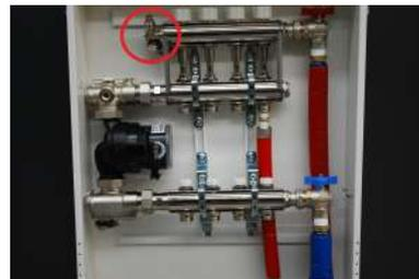
7. Filling the system: close the entry/return valves of the primary circuit (red and blue); open manually the first thermostatic shutter and turn the specific knob anticlockwise.
