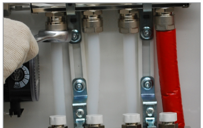
5. Connection and tightening of entry/return flow secondary circuit from high temperature and low temperature system
