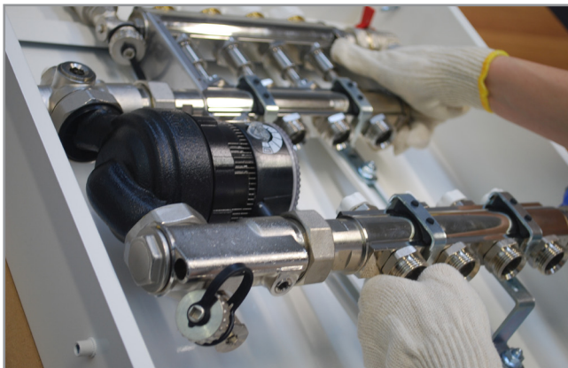
3. Install the control unit in the specific case, first releasing it from the top brackets and then from the bottom ones.
