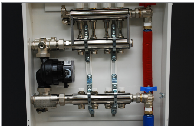
4. Connection of entry/return flow primary circuits from heat generator
