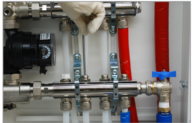
9. Filling the system: close the following lockshields by turning the Allen wrench clockwise
