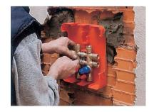
The connection of the pipe to the manifold begins, paying attention to the calibration of the end. The elements of the seal are inserted into the pipe: nut, olive and insert.
