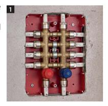
Example: 4x4 manifold installed and finished with activation of the valves by means of caps. Only the valves can be inspected and activation is always possible.
