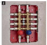
Example: 4x4 manifold installed and finished. It is possible to inspect the manifold and operate the valves after simply removing the door.
