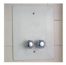
3) System with inspection of the manifold and valves: this is the most traditional system, always used in manifold systems; the two valves, incorporated in the manifold, can be operated only after opening the door.
