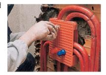
The chases are then grouted; at this point, a considerable part of the installation has been completed. The substrate necessary for laying the tiles will then be created.
