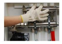
9. Filling the system: open the first lockshield by turning the Allen wrench anticlockwise.
