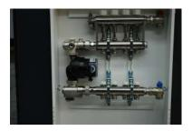
4. Connection of entry/return flow primary circuits from heat generator.
