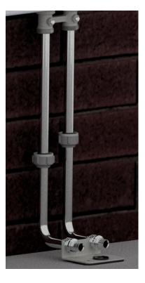
Manually screw the connection kits and mark the fixing point of the bracket with a pencil or marker.
